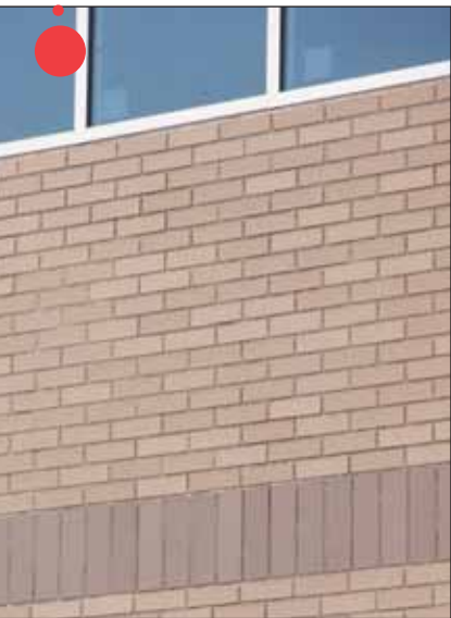
Brick inlays in concrete panel
