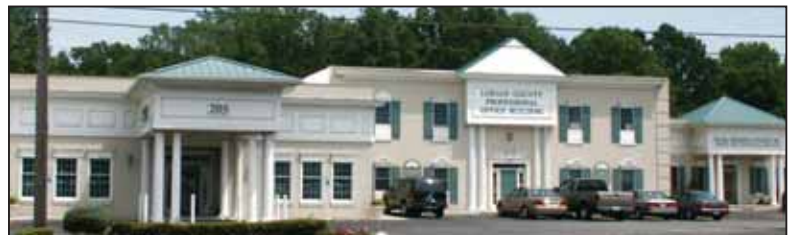
Stucco and pillars replaced the dated brick facade on these professional buildings.
