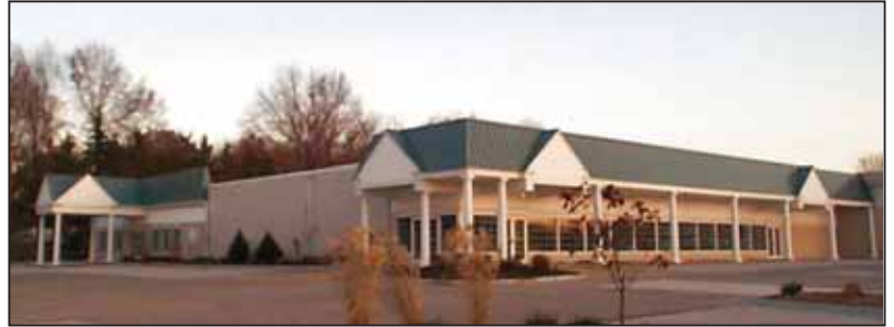
An old drug store was transformed into a sharp business center with individual tenant units.
